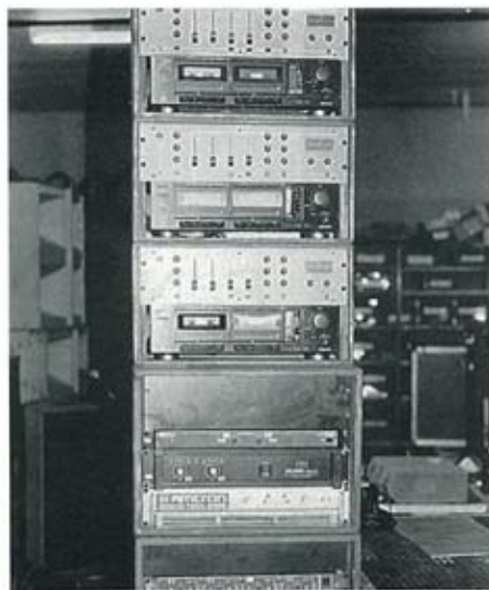
A stack of Games PA control systems ready to go on the road.
