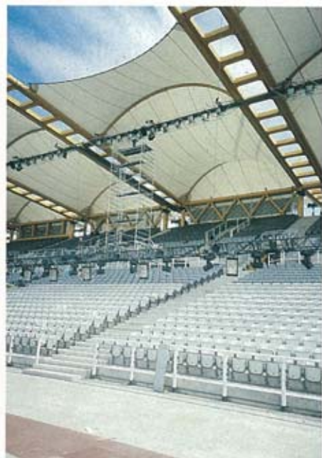
'Unusual' rigging the 80m lighting truss.
